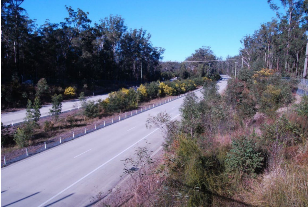
Pacific Motorway dissecting the flora reserve including the vegetated Island between north and southbound lanes. Note the fauna crossing 'ladder' and glider poles to facilitate fauna movement and mature blackbutt forest.
