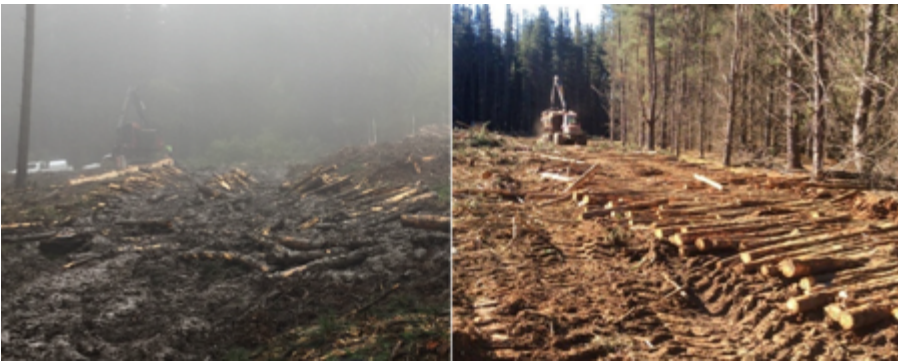
Figure 4.2 Use of cording and slash can prevent excessive rutting in wet weather
