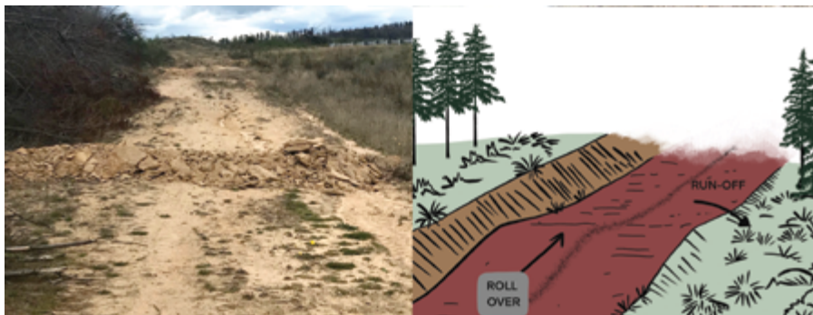
Figure 6.6 Constructed crossbank and rollover
