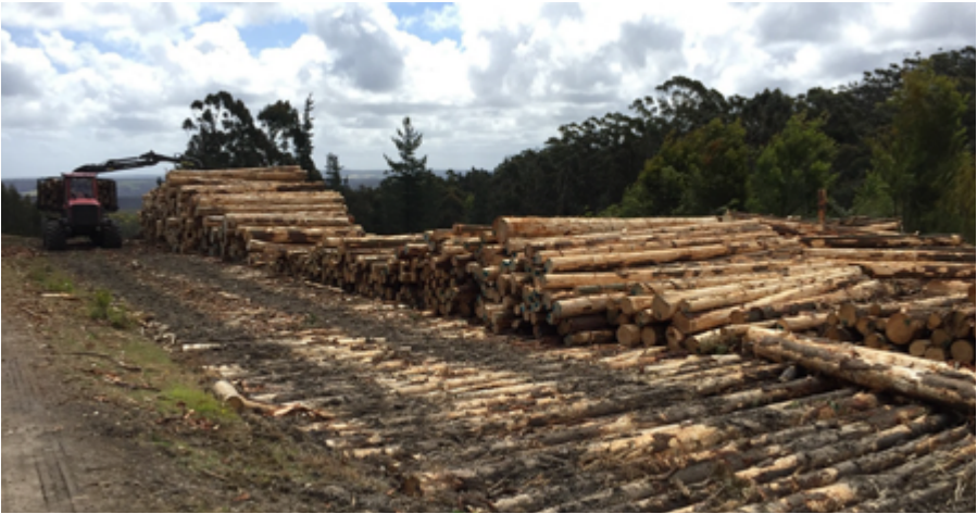
Figure 5.2 Cording used to minimise soil disturbance on the road verge
