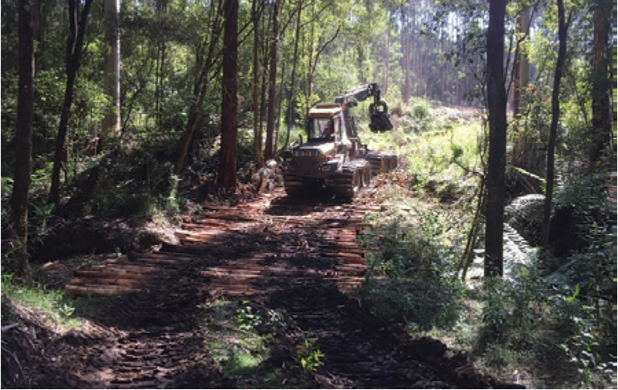
Figure 3.4 Drainage feature crossing must be approved and appropriately constructed
